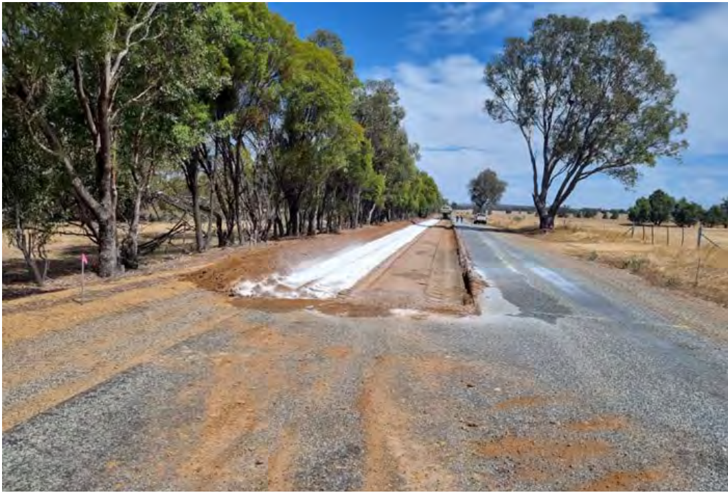
Lime Being Applied to the Section of Pavement
