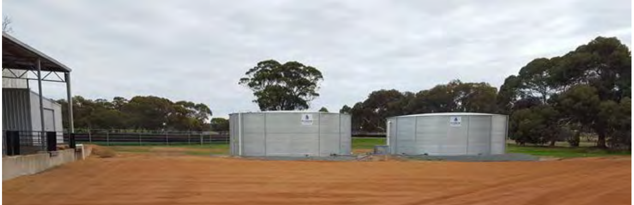
2 x 250kl Water Tanks Adjacent to the Ram Shed
