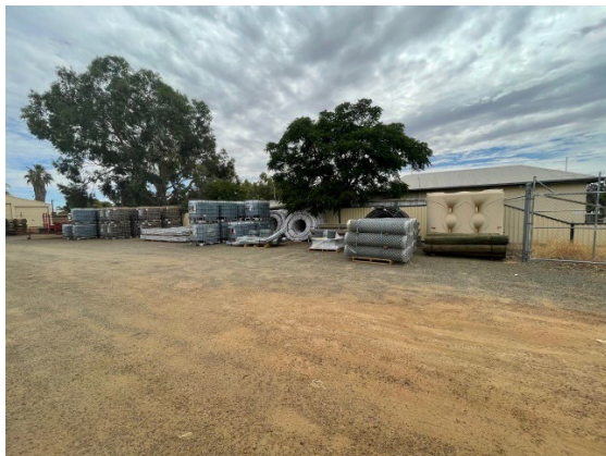
Figure 5: Delivery and Storage Area Facing Southwest
