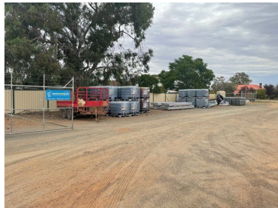
Figure 6: Delivery and Storage Area Facing Southeast
