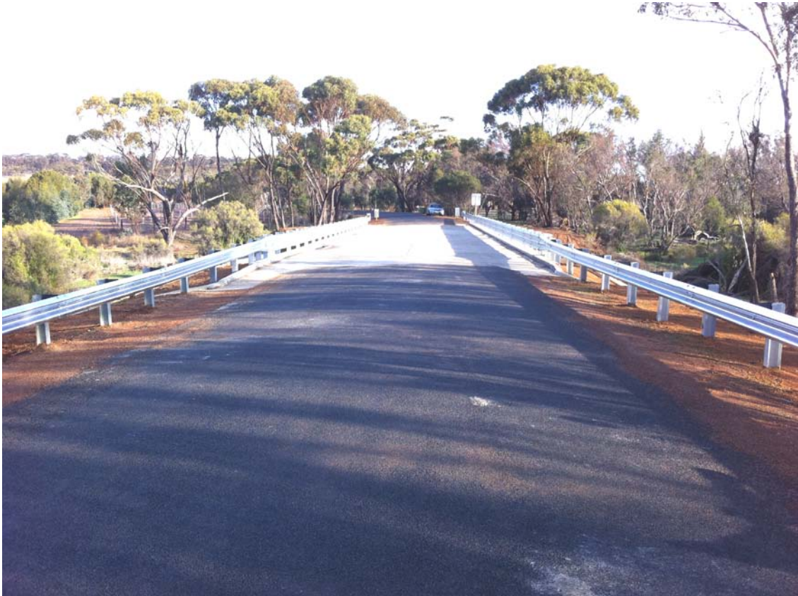
Photo – Clayton Road Bridge Widening & Resurfacing
