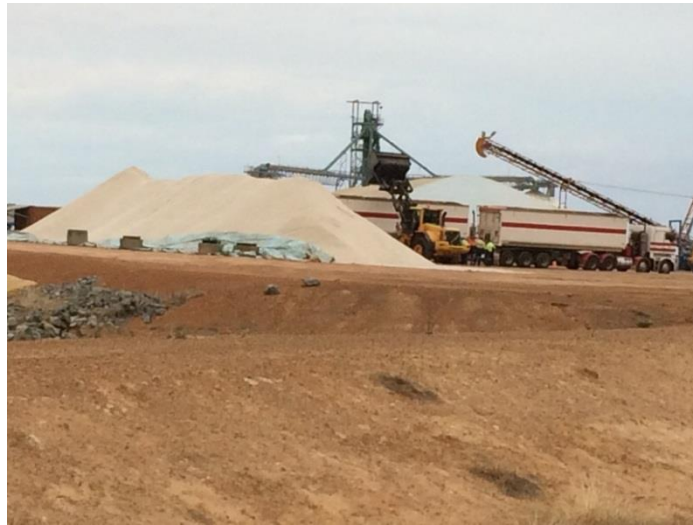
Loading from stockpile area
