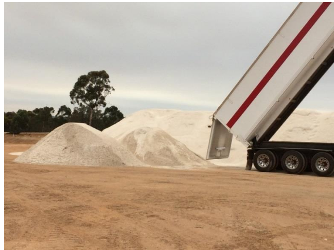
Delivery of stockpile area
