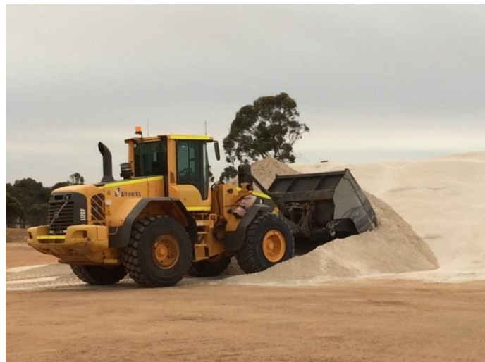
Loader pushing stockpile
