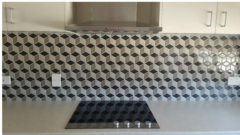
Kitchen splashback in one of the new units
