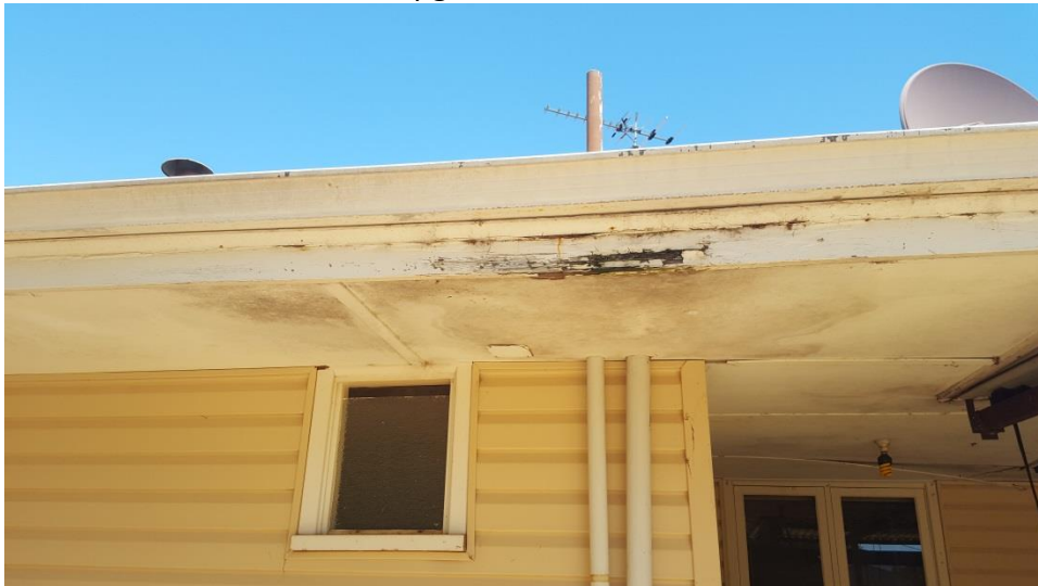
Painting eaves and exterior woodwork
