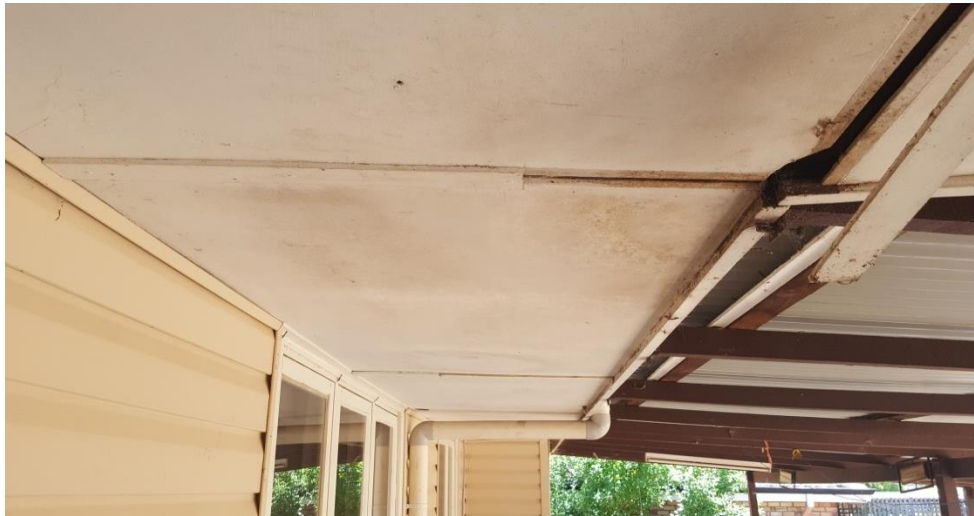
Rear patio repair
