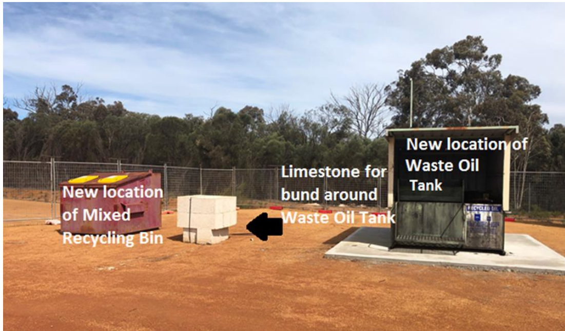
FIGURE 2 SHIRE OF WILLIAMS REFUSE SITE SEPTEMBER 2019, MIXED RECYCLING & WASTE OIL TANK RELOCATION.
