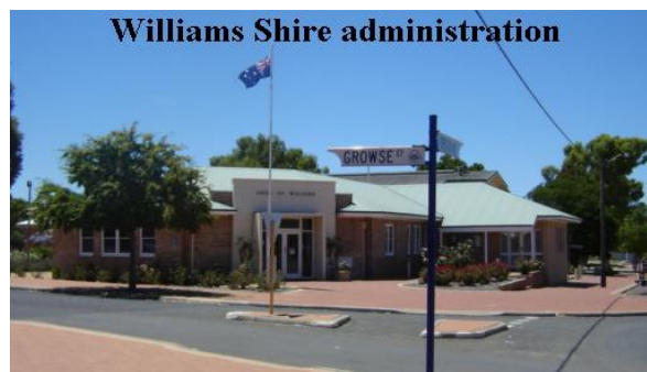
Figure 14: Paved pathways in front of Shire of Williams – cnr Growse Street & Brooking Street.
