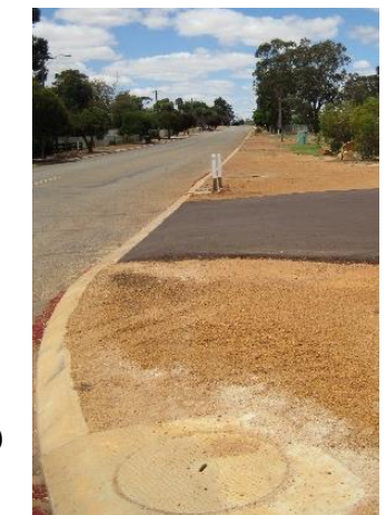
19: Richardson Street looking west to Albany Highway
