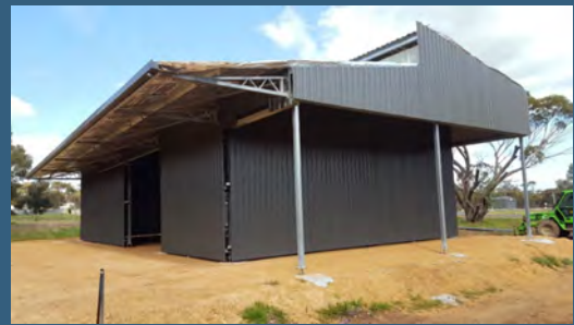
Williams Men's Shed Headquarters Under Construction
