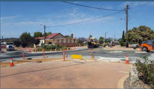
Asphalt installation on Brooking Street
